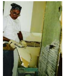
Ron Huffman tearing out a ruined wall.
